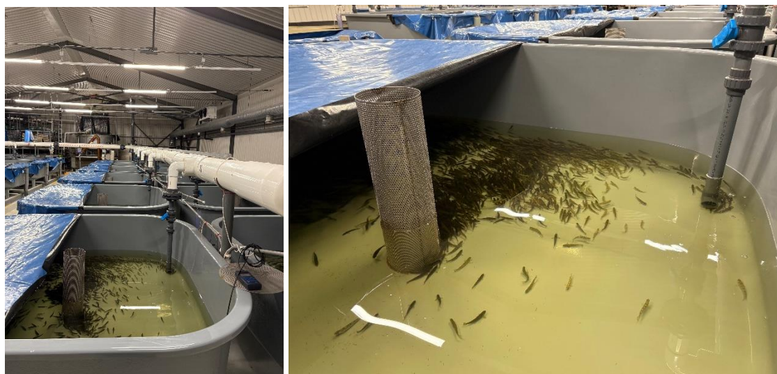
Fig. 1. Recirculating aquaculture systems (RAS) at the Eastern Region Pisciculture Division.
